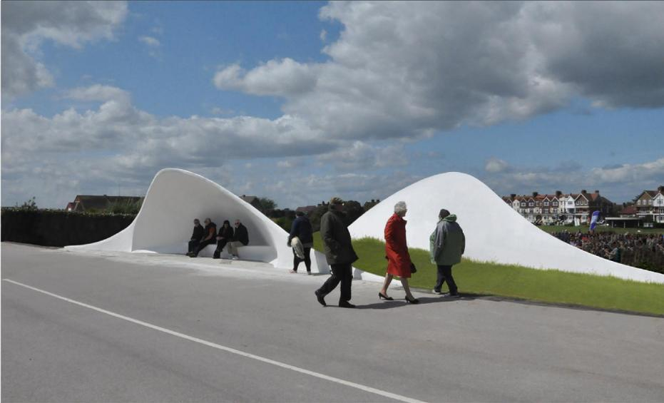
Built to a limited budget, Stage-by-the-Sea comprises two striking concrete shells that have been optimised for acoustic and structural performance. Sprayed concrete has been used to form the delicate shapes, yet still provide robustness. The material is acoustically perfect for focusing the music of performers using this community facility.
